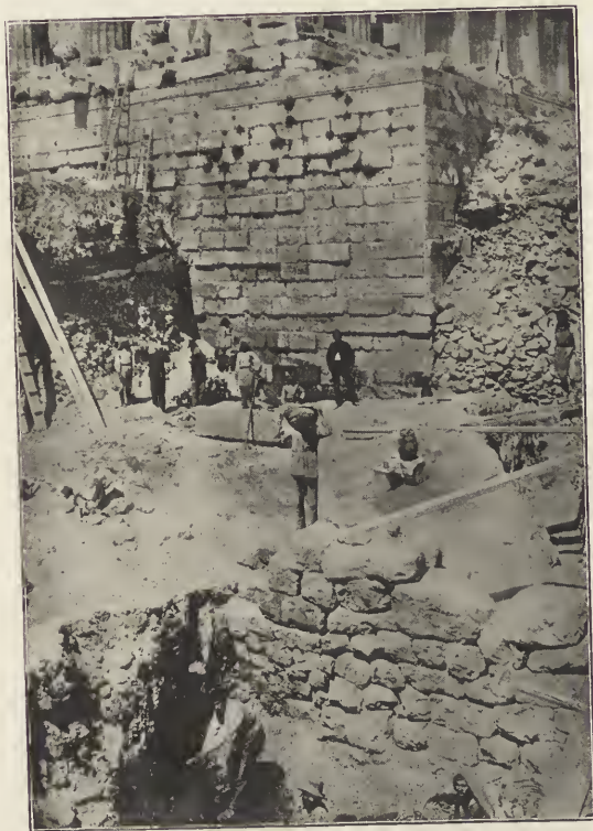
FIG. 28.—Southeast Corner of Parthenon, showing Foundations. Coarse Retaining Wall in foreground.
